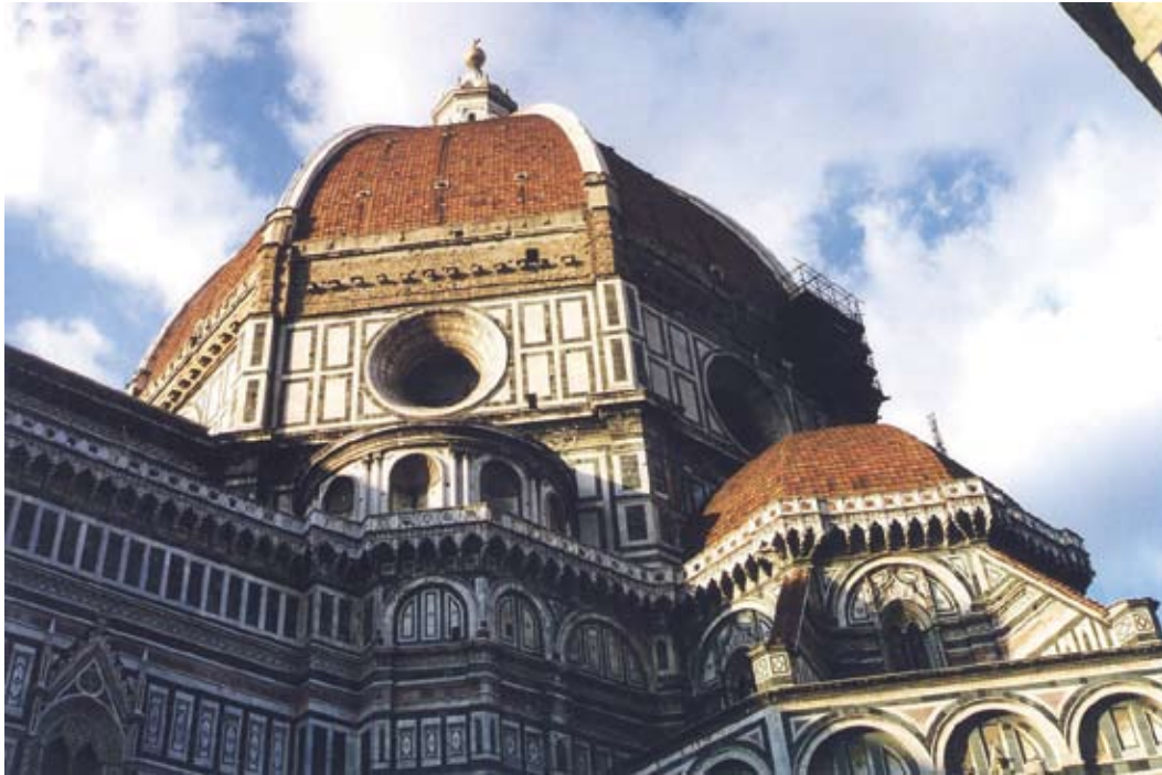
Brunelleschi's dome, the cupola of the Santa Maria del Fiore Cathedral in Florence, was constructed using the catenary principle.
