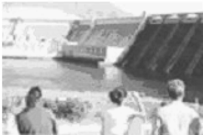
Here LYM members contemplate the magnificent construction of the Grand Coulee Dam.
