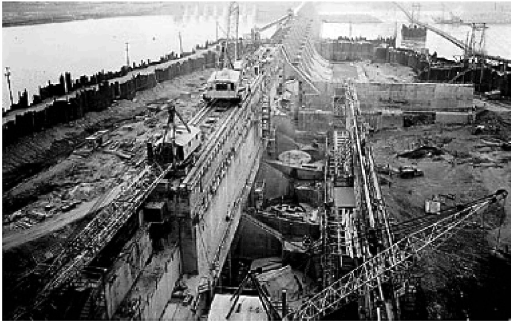
Construction of a dam and power plant by Roosevelt's Tennessee Valley Authority in 1942. Such state-organized public works can supply an effective degree of relative (Riemannian) physical-space-time curvature to the domain within which the relevant private enterprises are situated.
