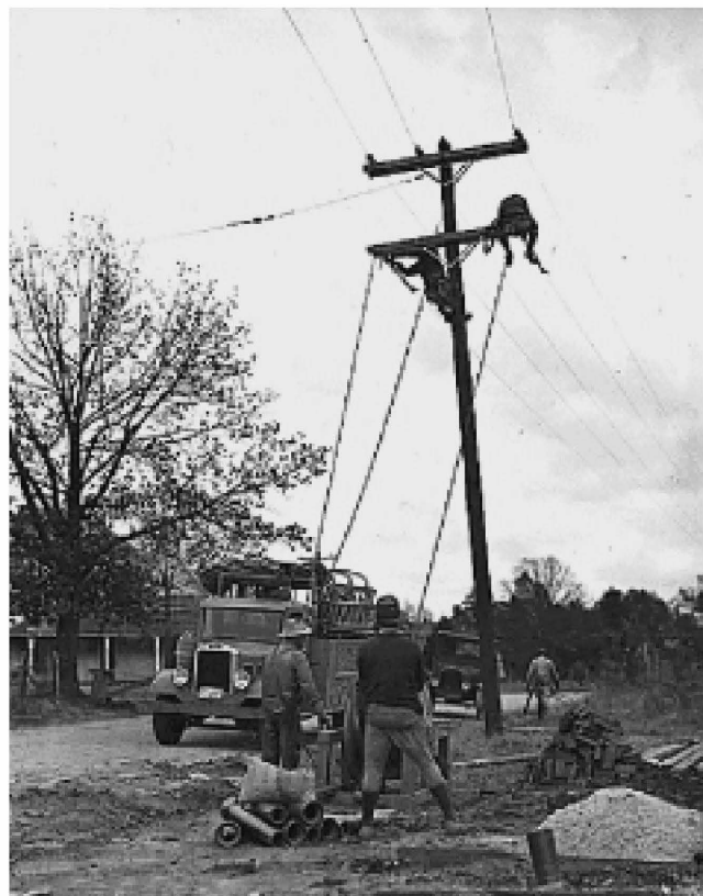
Franklin Roosevelt's Rural Electrification Act had incomparable effects on the productivity of U.S. agriculture. This shows electrical wire being strung in rural areas where the TVA was producing power.
