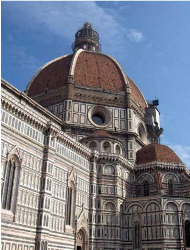
Filippo Brunelleschi (1377-1446) employed the catenary as a principle of physical geometry, for the construction of the cupola of Santa Maria del Fiore, in Florence, Italy. His statue is located within sight of the great dome.
